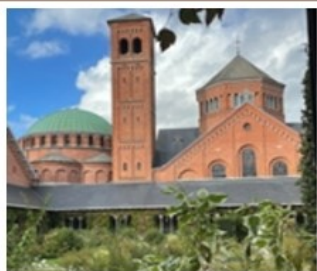
Cloister of St Andrew's Abbey, Zevenkerken-Brugge
